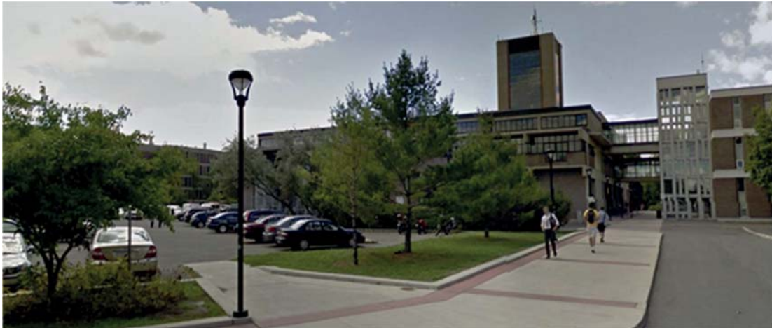
Figure 6. Architecture Building east façade, 2018
