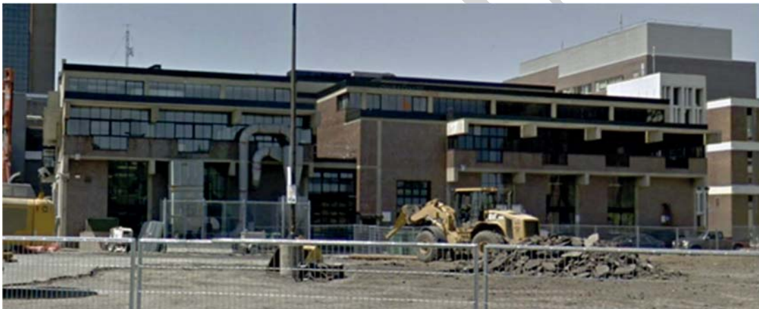
Figure 4. Architecture Building east façade, 2018 – Starting of construction phase
